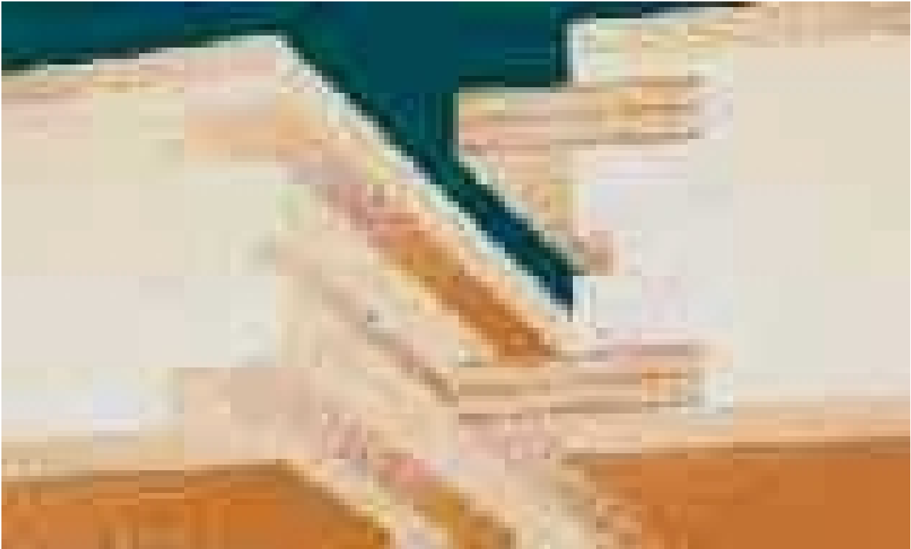
Figure 3. Cross-section through OSB 3 spline connection.
